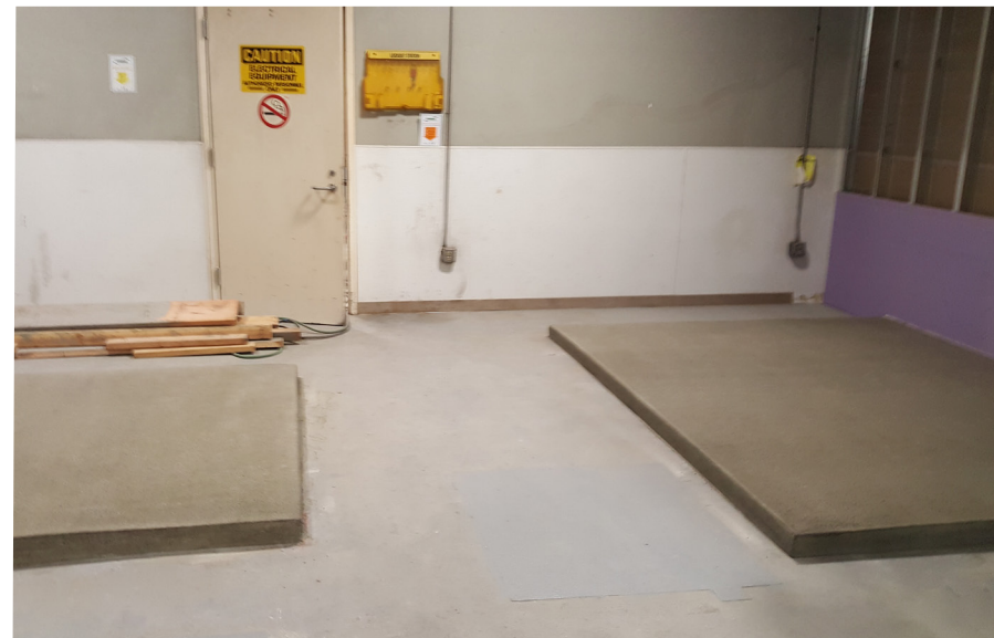
Stellar retrofitted this small existing space to accommodate a boiler addition including water treatment system. We updated the ventilation system to adhere to code compliance and added the equipment pads. Additional skid-mounted equipment was configured for installation in this same space. The new equipment provided support to the existing facility mechanical systems with seamless integration and virtually no loss to plant production output.
