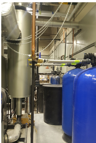
Stellar retrofitted this small existing space to accommodate a boiler addition including water treatment system. We updated the ventilation system to adhere to code compliance and added the equipment pads. Additional skid-mounted equipment was configured for installation in this same space. The new equipment provided support to the existing facility mechanical systems with seamless integration and virtually no loss to plant production output.
