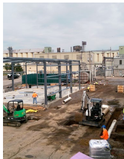
ERECTION OF PEMB BEGINS AT WEEK 15
