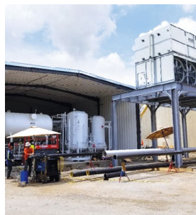
PACKAGED UNITS ARE INSTALLED
