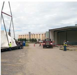
PEMB IS READY FOR PACKAGE INSTALL
