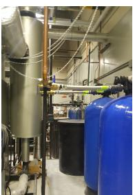
Stellar retrofitted this small existing space to accommodate a boiler addition including water treatment system. We updated the ventilation system to adhere to code compliance and added the equipment pads. Additional skid-mounted equipment was configured for installation is this same space. The new equipment provided support to the existing facility mechanical systems with seamless integration and virtually no loss to plant production output.
