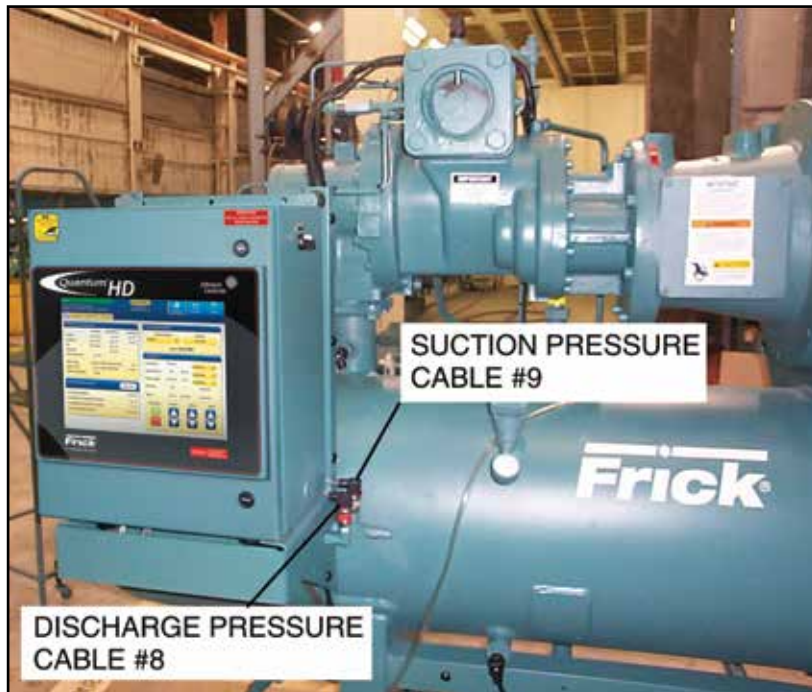
Figure 28a. Wiring Harness Installation, RXF 58 – 101.
