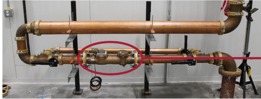
*This client decided to add a flow-meter to their water supply after installation of domestic water piping. Stellar's solution to accommodate the request was a redesign of the piping that was engineered and installed in one day.*
